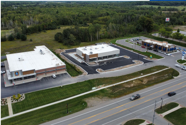
Started in Early 2022 the newest addition to the DDA district is the New Starbucks Plaza that will include two other store fronts and connection to the sidewalk for increase pedestrian access.
